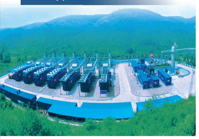
Gensets can be operated with natural gas, biogas, landfill, sewage, and coalmine gas as well as a wide variety of special gases.
